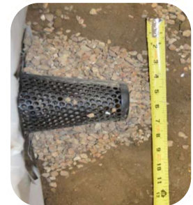
#57 stone packed around filter
