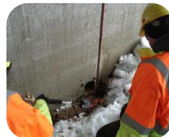
Creating access by clearing snow with torch
