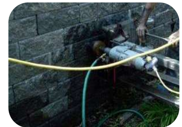
Core drill with water supply
