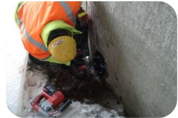
Using cordless tools to mount Jet Filter cartridge
